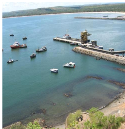
Marine structures Ports Jetties Coastal Structures
