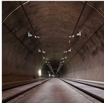
Concrete roads and food paths
